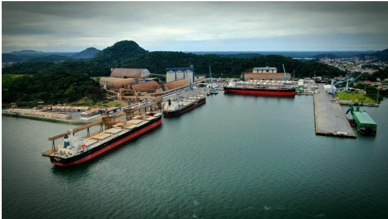
The São Francisco Port aerial view.
