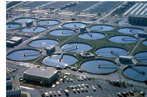
Sewage and Water treatment
